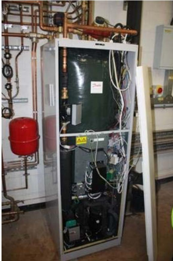
When treated (aerated) water used, heat exchanger and filter rapidly became clogged
